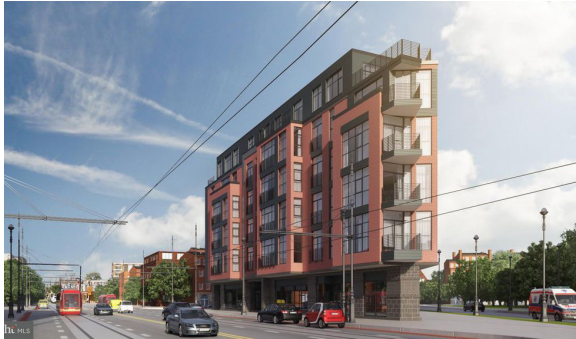
Housing and infill development: Newly constructed property at 1402 H Street NE, Washington, DC
