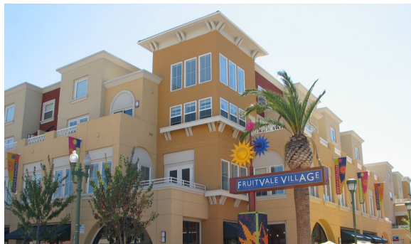
Fruitvale Transit Village, Oakland, California
